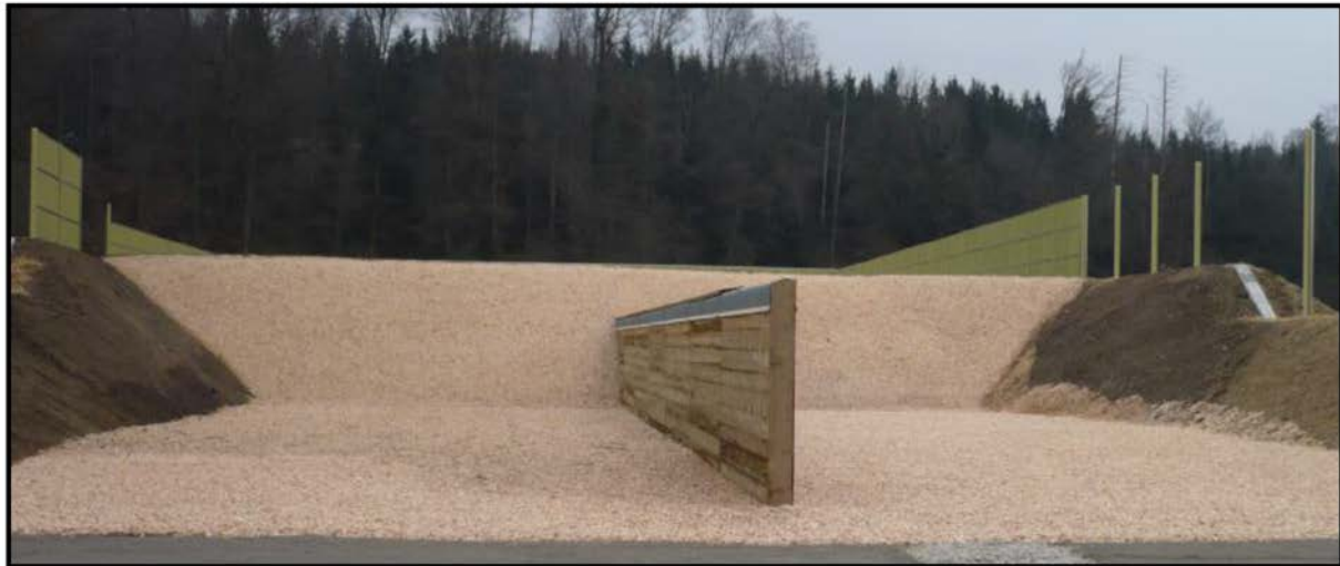
Figure 6: Standard short distance range in Switzerland with a complete cover of woodchips to prevent ricochets. The green structures are noise barriers.
